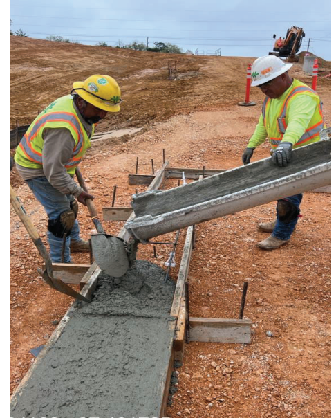
WTP – Drive 2 Placing Ribbon Curb
