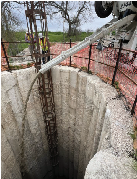
Seg D – Receiving Shaft CLSM Backfill
