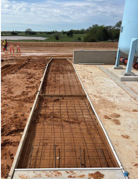
WTP – Setting Form & Wire Mesh for Sidewalk
