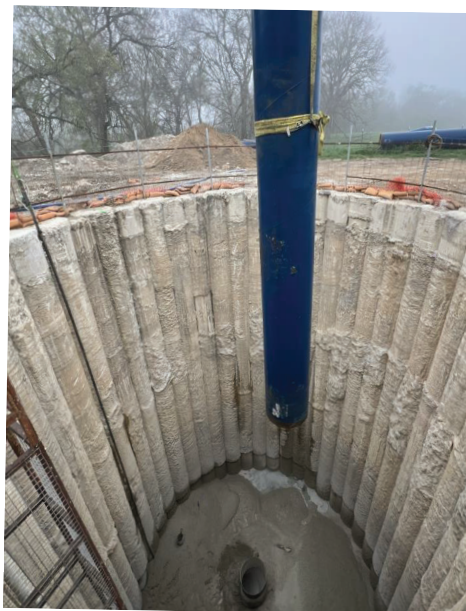
Seg D – Vertical Pipe Placement
