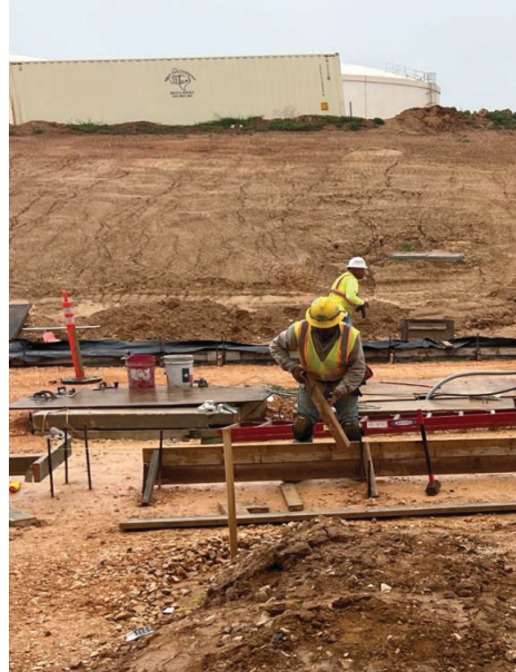
WTP – Drive 2 Setting Forms for Curb
