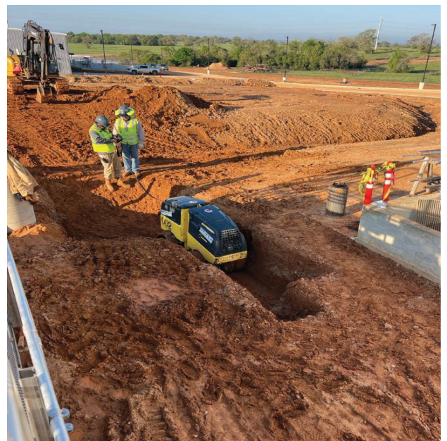
WTP – Backfilling Ground Wire Trench Between Rapid Mix and Lime System.
