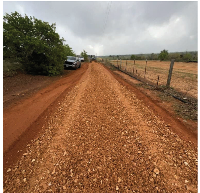
Seg A - Installation of Road Base at Rifle Road
