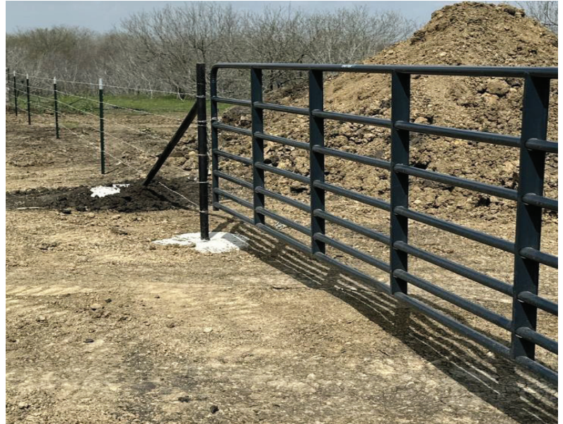
Segment B – Completed Fence Gap East of Tower Road
