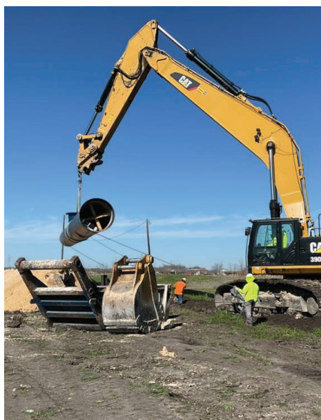
Seg E – Moving Pipe into Position to Lower
