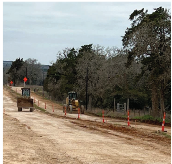
WTP – Grading Sides of Wolf Run Road
