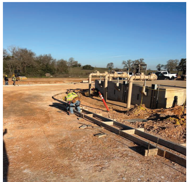
WTP - Drive 2 Setting Ribbon Curb Forms
