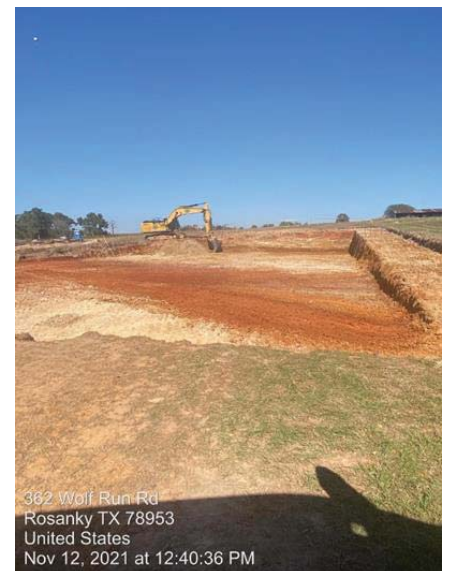
WTP/RWI - Filter Complex excavation
