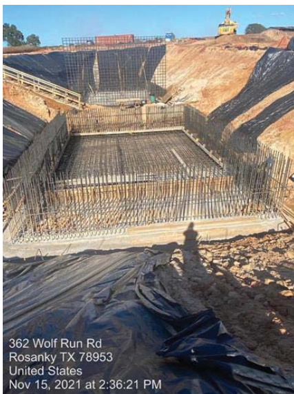
WTP/RWI - Recycle Pump Station
