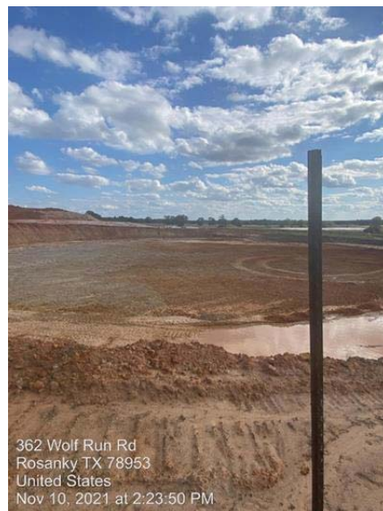
WTP/RWI - Clearwell excavation
