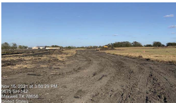
BPS – Clearing for Access Road
