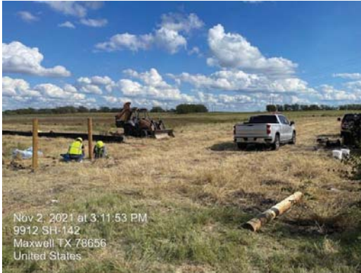
BPS – Placing fence and gate at entrance
