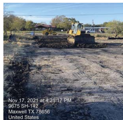
BPS – Construction entrance preparation
