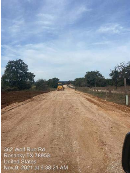
WTP/RWI - Temporary Access Road
