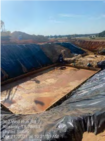
Recycle PS mud slab & formwork
