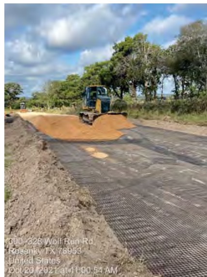
Temporary Access Road base
