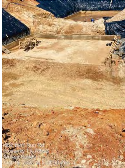
Recycle PS mud slab & formwork
