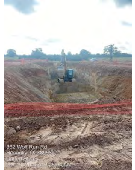
High Service PS excavation
