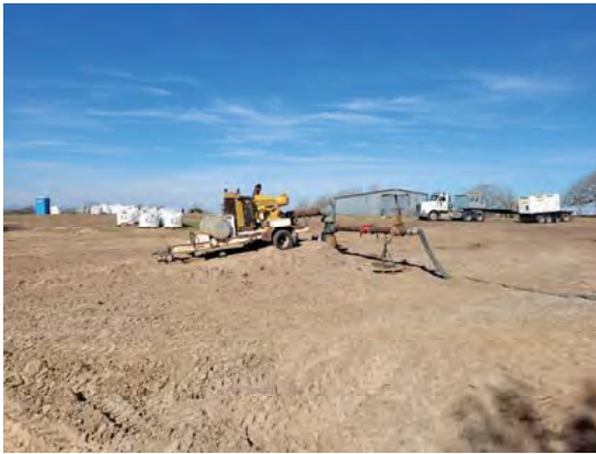
Well No. 6 Pumping for Development
