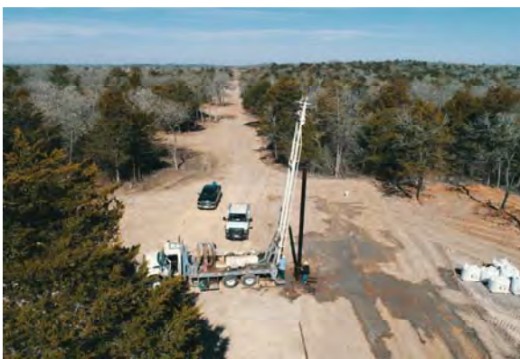
Well No. 7 Bailing for Development
