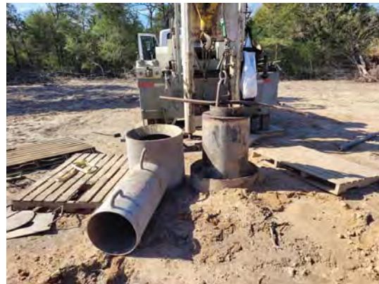
Well No. 7 Bailing Discharge
