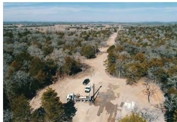
Well No. 7 Bailing for Development
