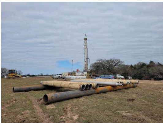
Well No. 6 14-inch 304 SS Pipe-based Screen
