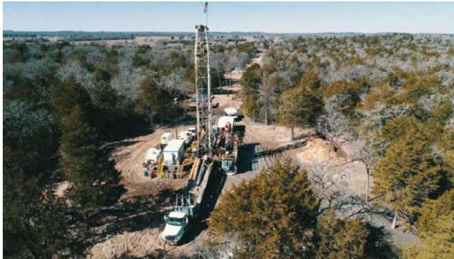
Well No. 7 Screen Installation
